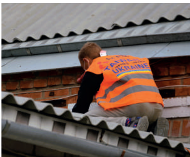
Roof repair in Tsyrykuny
